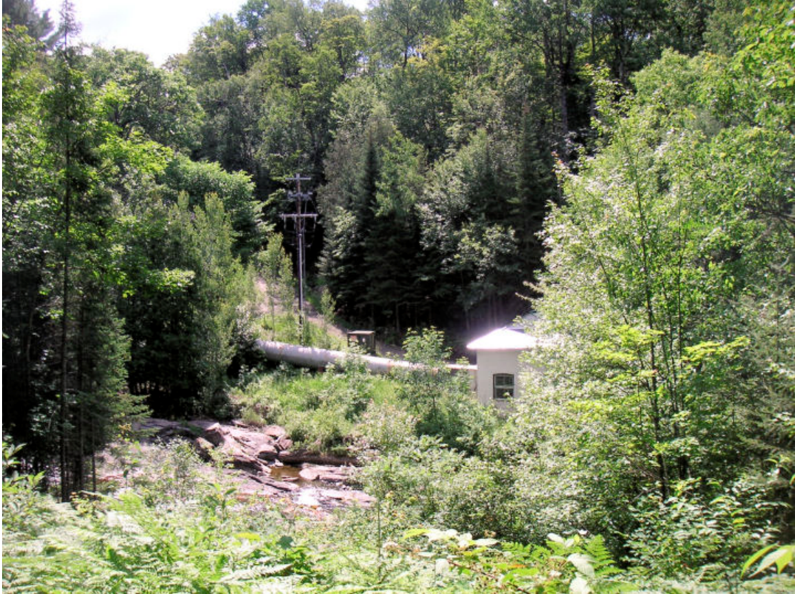
View of power generating station below dam, showing water inflow pipe, and the first electric utility pole used for transmitting generated power to the grid.
