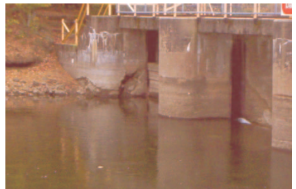
Dams are deteriorating and in serious need of repair. Logs provide only crude control of water levels.
