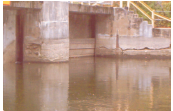
Dams are deteriorating and in serious need of repair. Logs provide only crude control of water levels.
